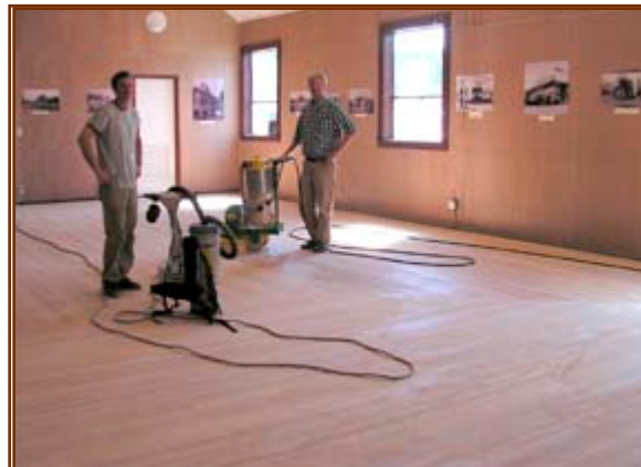
Lynch Brothers Hardwood Floors recently took on the big task of refinishing the floor in the main hall of Leedy Grange. The old-growth fir floor hadn't been worked on in about 30 years, and stains and holes made it a tricky job. They're still putting on the finishing touches, but the Grange is looking forward to welcoming dancers and parties to our spiffed-up hall. Information about Leedy, including rental policies and rates, is on the website at leedygrange.org
