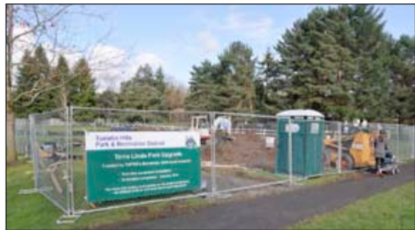
Terra Linda Park playground under construction. Photo by Neil Hefty
