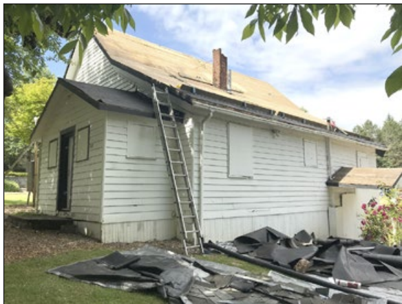
The new roof is going on to the JQA Young House. Soon the 1860's building will also get a new coat of paint and new windows and doors!
