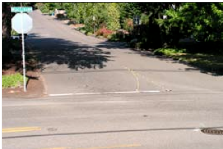
NO LEFT TURN: An arrow and the word "ONLY" will be painted on the pavement and a no left turn symbol sign will be installed under the existing stop sign. Advance warning signs may be added later if needed.
