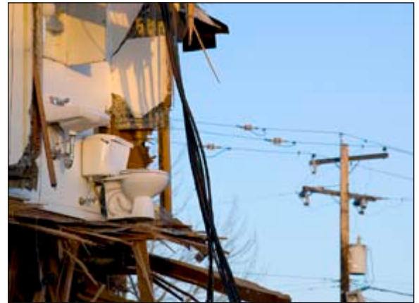
Cedar Mill News photographer Neil Hefty caught a humorous moment when the apartments were being demolished
