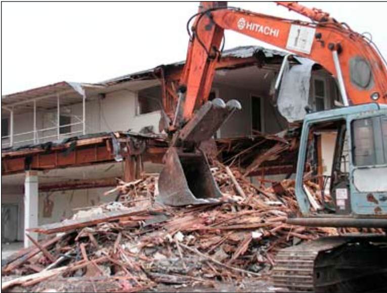
Northwest Earthmovers' skilled demolition workers carefully sorted the piles of debris so that most of it could be recycled—the wood will be made into chips, and the metals are sorted and distributed to area recyclers.
