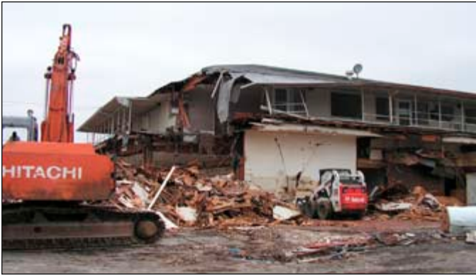
Demolition on the building started at the back.
