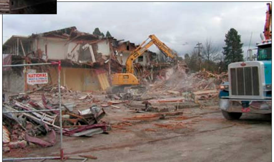
Load after load of debris was hauled away during the two-week demolition process
